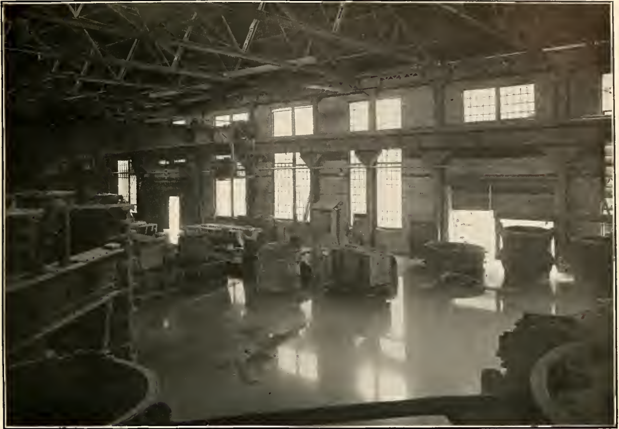
FLOOD OF MARCH 15, 1907. One of the large manufacturing plants.
